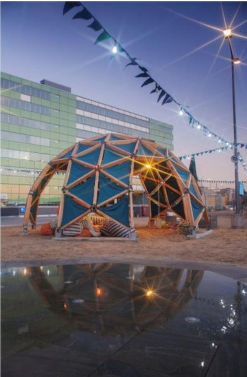
**GRID-7-4** is a geodesic dome with wooden frame and steel connectors. It is an amusement pavilion or temporary shelter.
